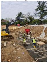
1500 geo-piers were placed in the ground to support the building and contaminated materials were excavated and placed in their secure locations. Over the last several weeks – we now have a pool!....sort of. From the attached pictures you can see the 50 meter pool basin has been excavated (you can see the deep end, the slope to the
