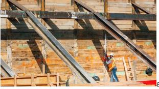
support of excavation (SOE) system to provide temporary structural support for the jobsite during mass excavation. The project's temporary SOE system – a combination of steel support posts,
