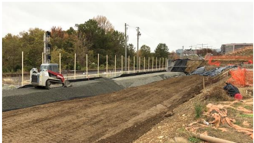
Building the Esplanade: The raised pathway sits on soil dug up to create the adjacent ballfields. The Esplanade was not part of the county's original plans for the park.
