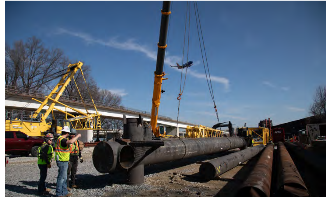
Crews preparing pipes for pile driving
