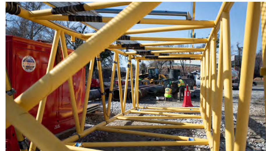
Crews preparing pipes for pile driving.
