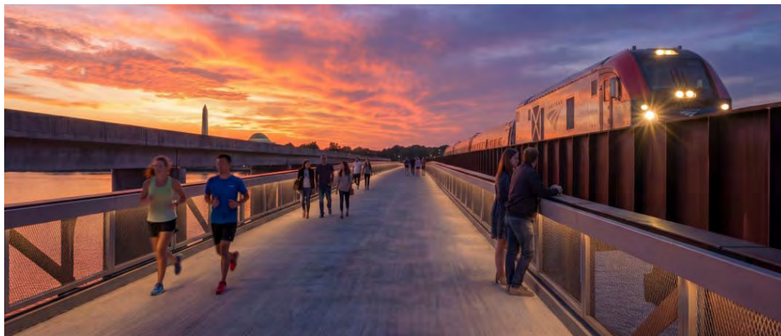
New Bike-Pedestrian Bridge: 16 ft wide
