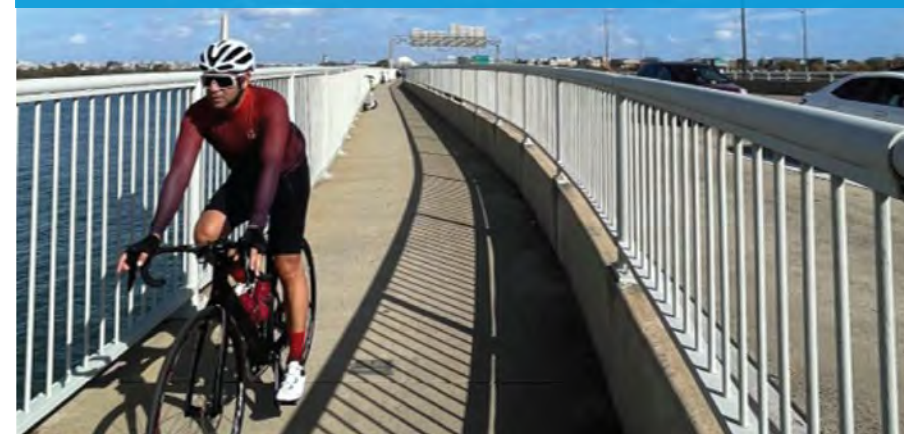
Existing 14 th Street Bridge Bike-Ped Path (7'-6" width)
